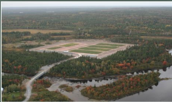
Appleton/Glenwood Wastewater Treatment Facility
