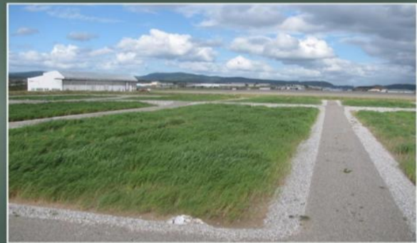
Stephenville Wastewater Treatment Facility
